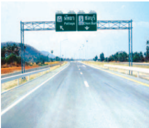
泰國曼谷-Chonburi New Motorway
