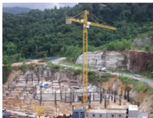
Construction of 28-storey Coastal Tower Condominium, Penang
