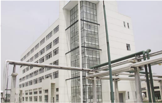
The GMP Transformation Shop of Hutchison Pharmaceutical, Shanghai
