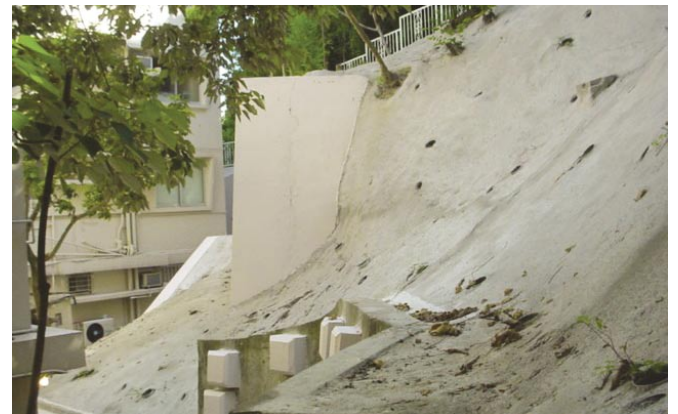
45 Sassoon Road, Hong Kong
