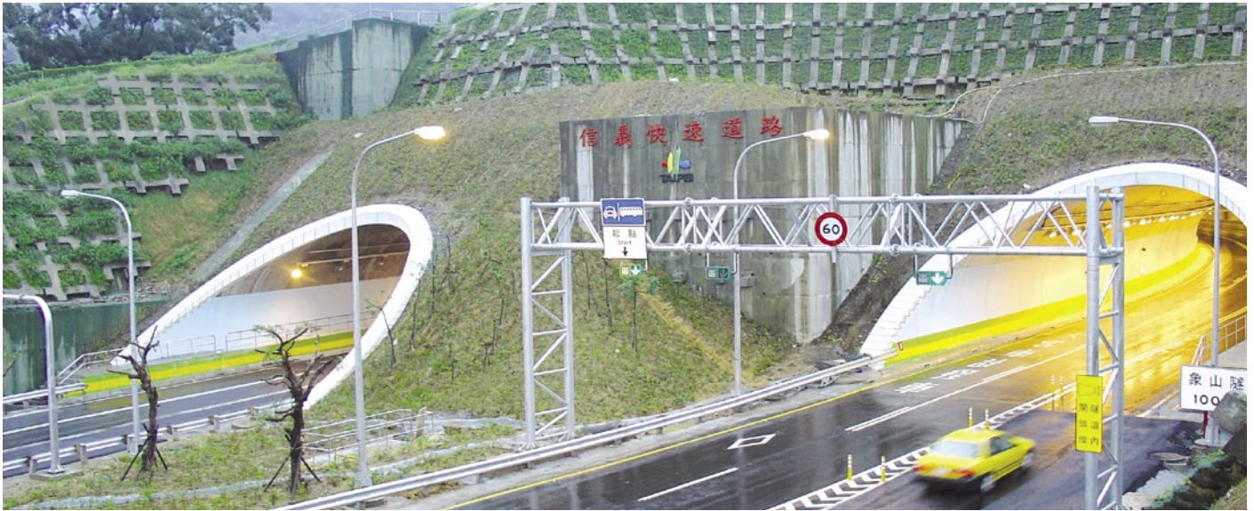
Xin-Yi Expressway Tunnels
