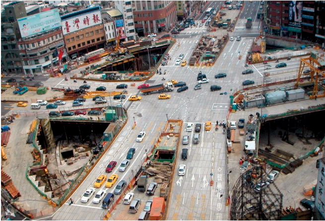
Largest self-circular diaphragm wall in the world during construction.
