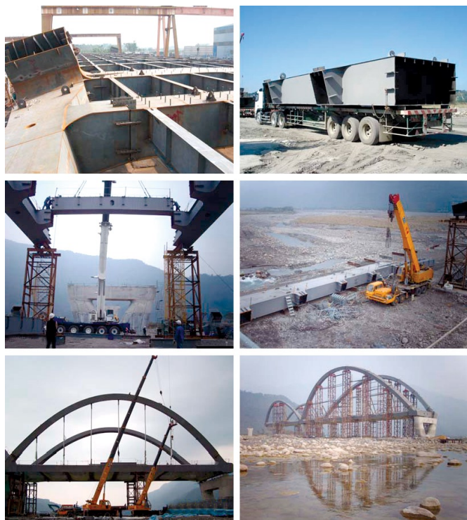
Sinwei Bridge during construction
