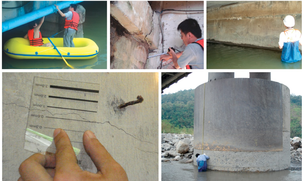
Visual Inspection of Township Bridges of Yilan County
