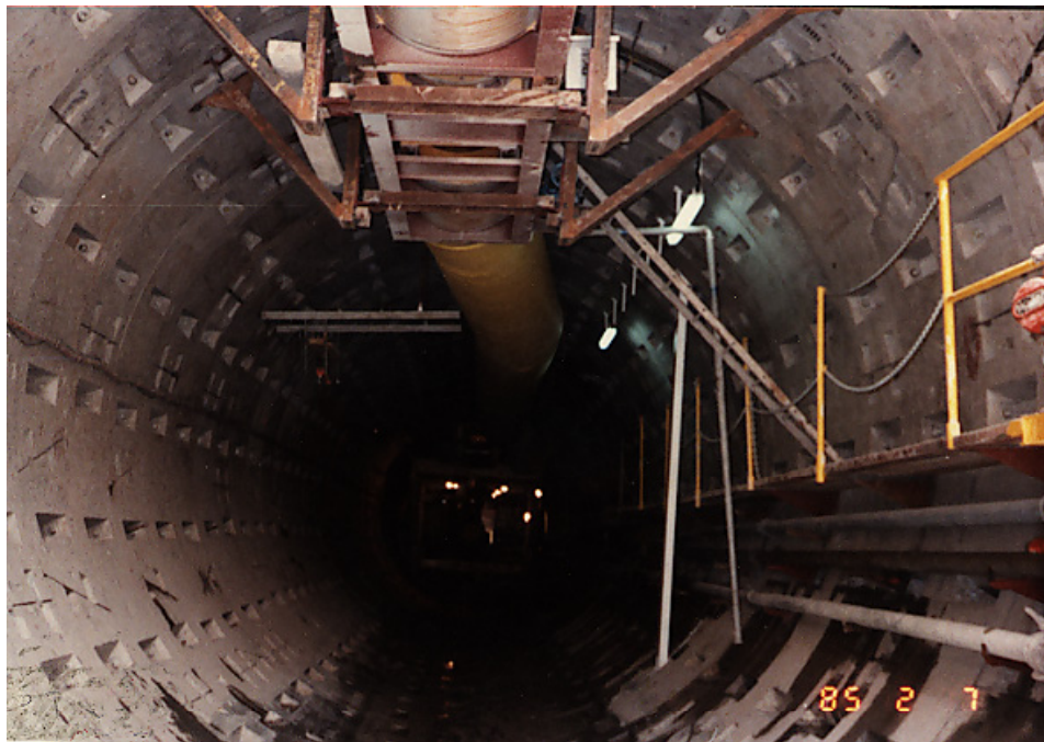
Figure 2 Reinforced Concrete Lining for a Tunnel
