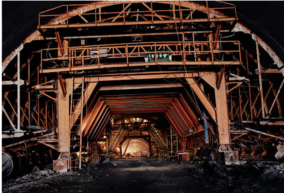
Figure 1 Temporary Supports to a 4-lane Road Tunnel ( Courtesy of RESA Engineering Corporation)
