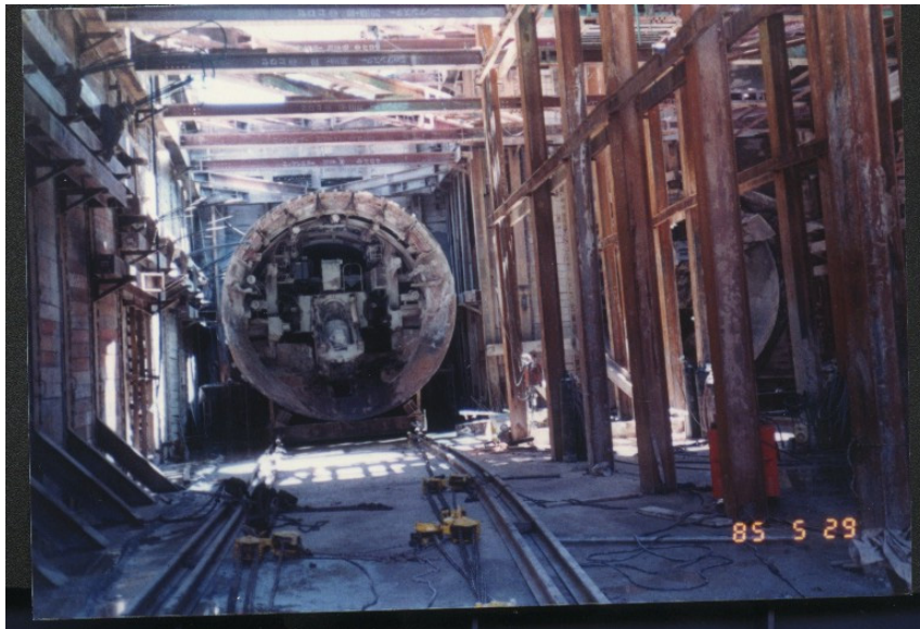
Figure 2 Arriving of a shield tunneling machine at a station
